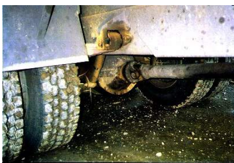
Figure 1. View of the truck suspension system
